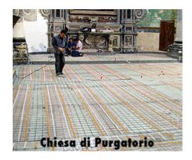
For the areas where it is not possible to lay new floor company SCARPA s.r.l. developed the new system called "Terra Plate" (see pictures bellow). That systems is composed of insulation layer, heating film ECOFILM, covering PE foil and the floor covering. For the fast warming up there is used the heating film with surface output 300W/sqm with floor sensor to avoid the surface floor temperature will exceed 30°C.
