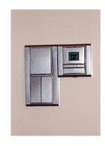
Regulation of the floor heating is provided using programmable room thermostats with floor probes.
