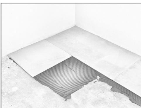
When affixing the boards onto a wooden foundation or other foundations that are unstable with regard to their dimensions, the adhesive sealing cement must be sufficiently flexible. For that purpose, we recommend using the 10 mm F-boards. For these foundations, we recommend anchoring the boards with at least 4 anchors per board and placed at least 30 mm from the edge of the board.
