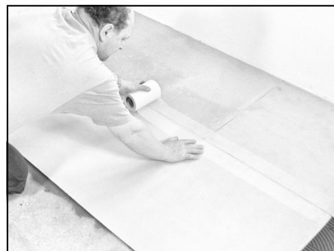
The spaces should be covered with a reinforcing gauze fabric tape. Place the tape, apply flexible sealing cement, spread the residual material with a spreader or remove it. The tape should overlap at least 50 mm. Allow the adhesive material to harden, as described in the instructions for use.
