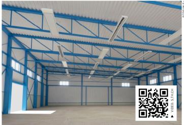
► ECOSUN S+ / S+Anticor – for industrial halls, gyms, halls, workshops, with a rating that corresponds to the given environment. Suitable for drying of buildings. For spaces with higher humidity – agricultural structures, washing facilities, panels are produced in a corrosion-proof version S+Anticor.
